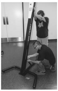
**13.** Then go back and TIGHTEN FULLY the <u>TOP</u> lock nut on the tubular brace.
